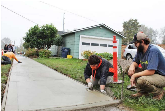
Nichole Rose joints the concrete.
